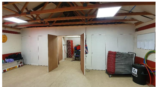
New cupboards in the hut have been completed
